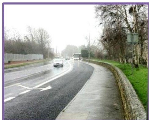
Surface Upgrade of Bus Route
