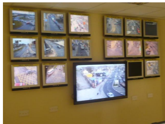
Traffic Control Room
