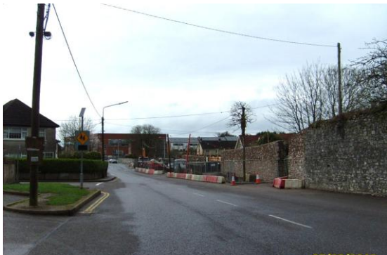
Boreenmanna Road – under construction
