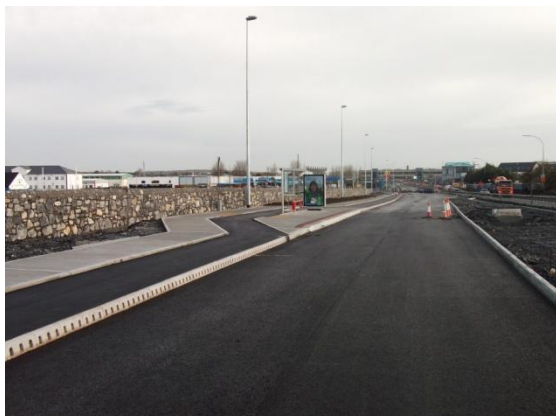
Seamus Quirke Road Scheme (Under Construction)
