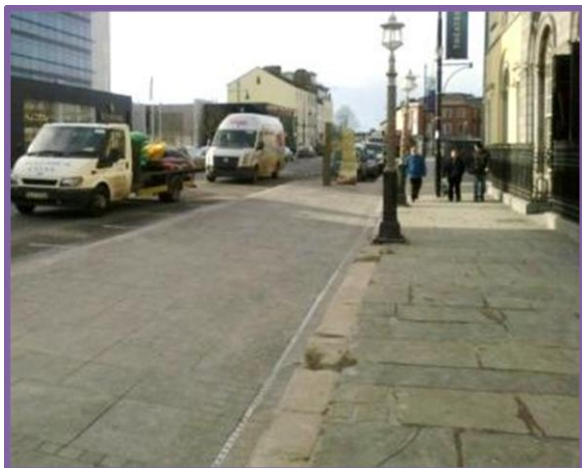
South Quays Green Route – Widened Footpath
