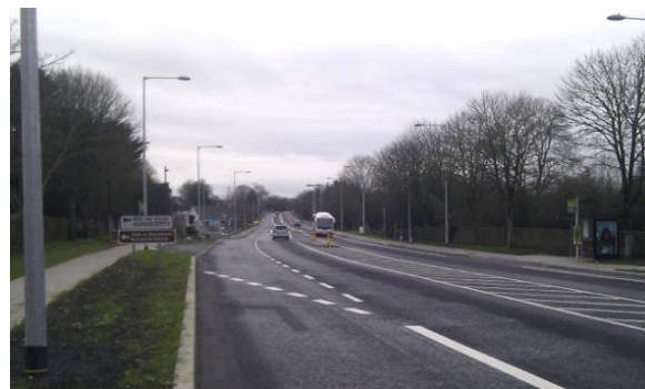
R445 Dublin Road Green Route Phase 2
