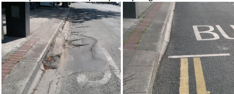
Blackrock QBC opposite St. Vincent's hospital – before and after works.
