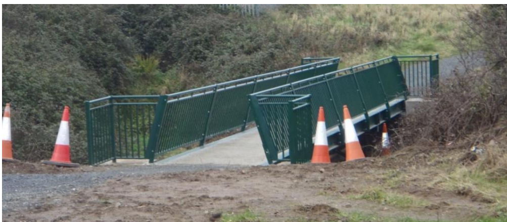
After - Cliff Walk footbridge
