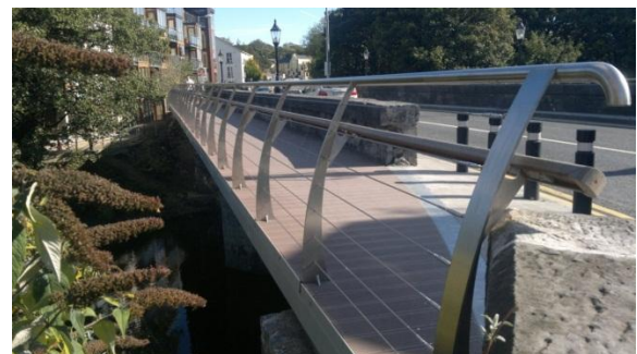
New cantilevered footpaths.
