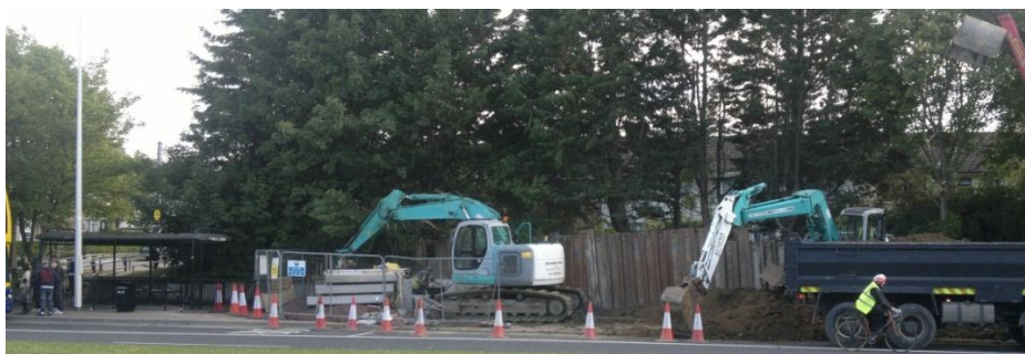
N11 Inbound, Stillorgan during construction
