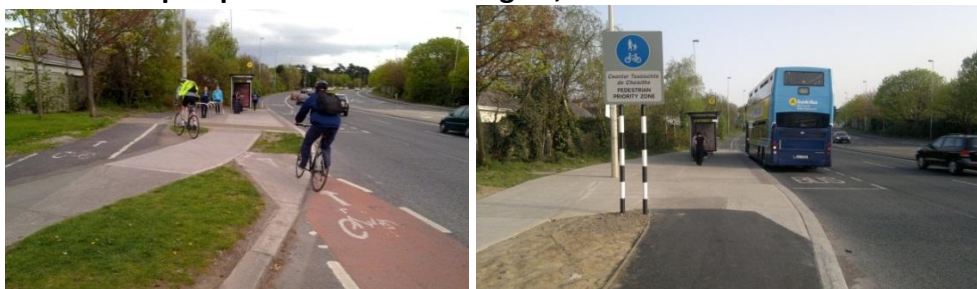
N11 outbound, Stillorgan – before and after works.
