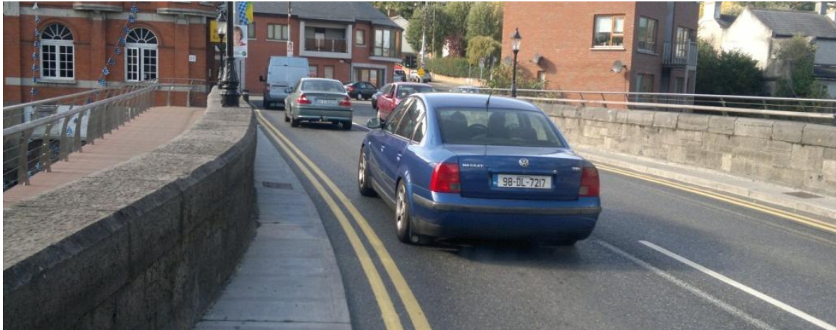
Bridge with original narrow footpaths.
