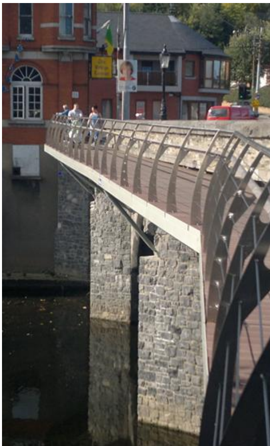
New cantilevered footpaths.
