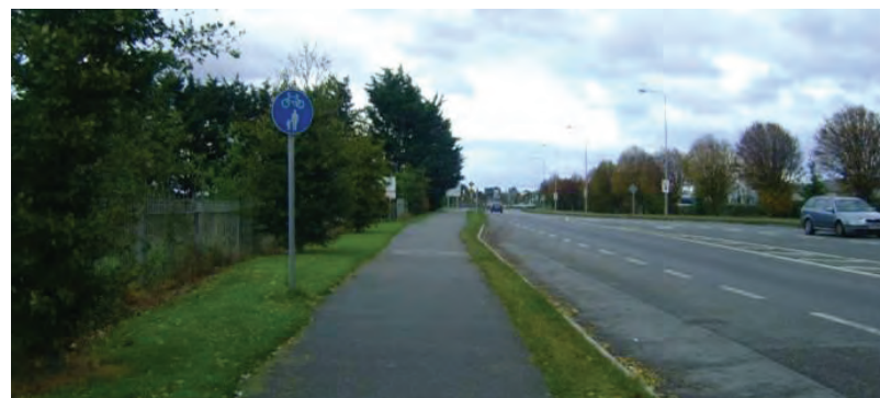
Existing Shared Pedestrian and Cyclists Facilities on Dublin Road, Naas
