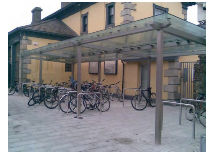
High quality and well located cycle parking shelter at Greystones DART station
