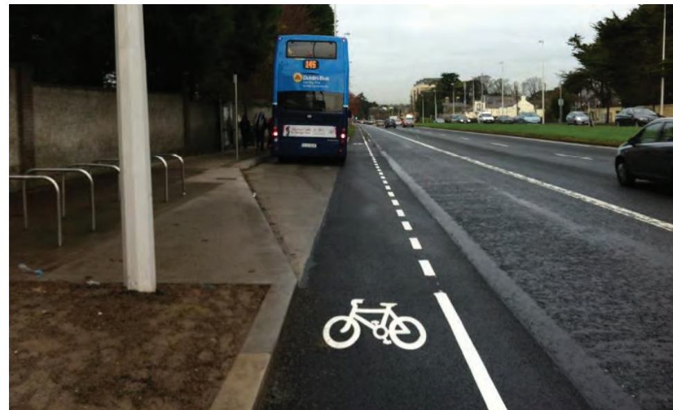
Recently upgraded Cycle Lane at Bus Stop on N11
