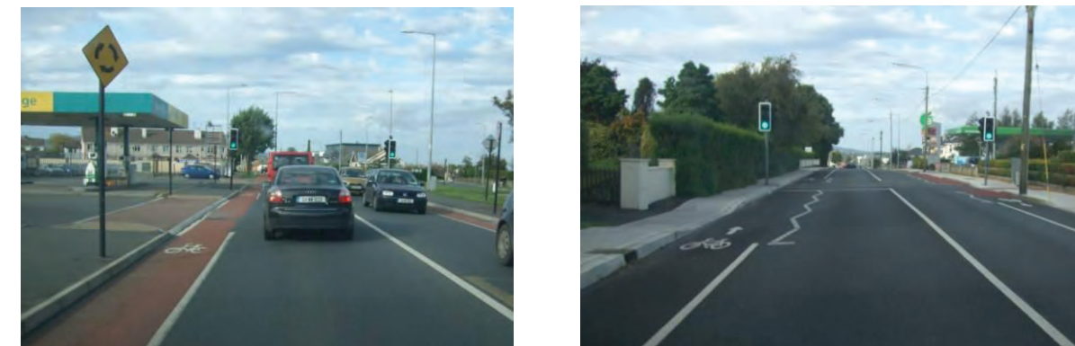
Existing Cycling Facilities on the R772 Wexford Road, Arklow
