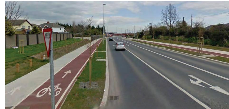
Existing Cycle Tracks on R114 Firhouse Road
