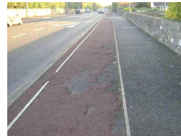
Existing Cyclists Facilities on Straffan Road, Maynooth
