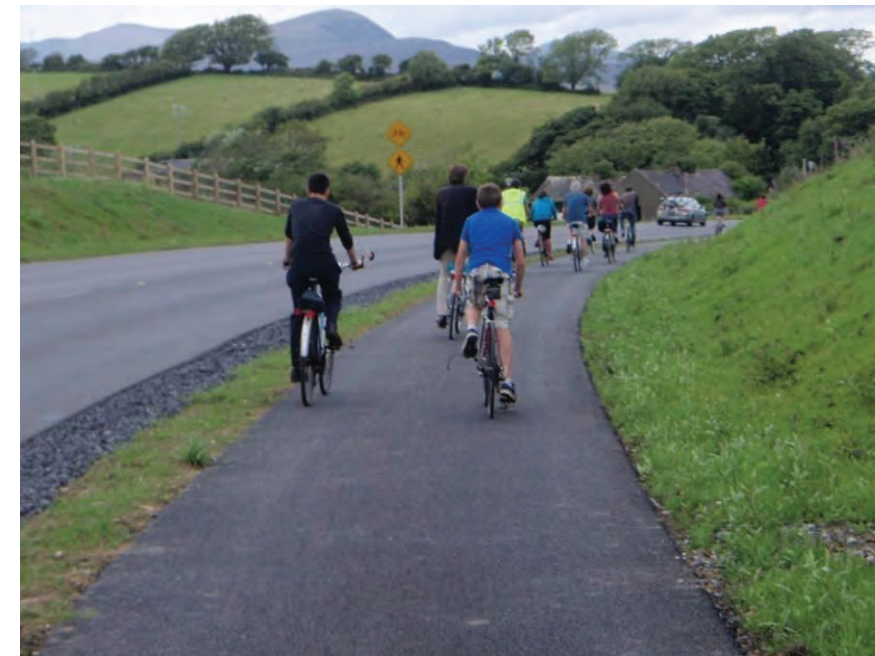
Cycle Track alongside the N59 at Newport, County Mayo
