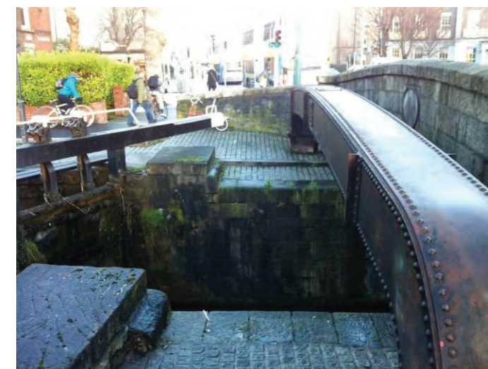
Leeson Street Bridge - Western side
