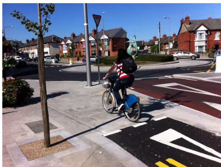
Cyclist using shared space on new roundabout
