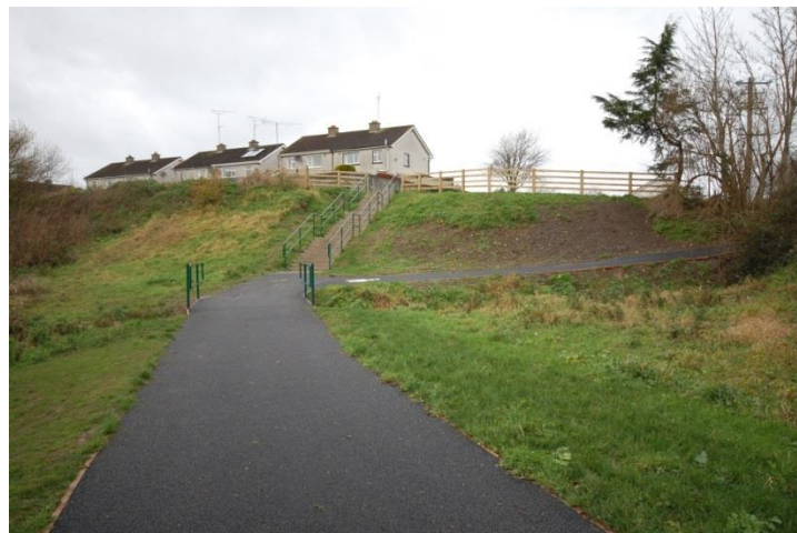
Widened and resurfaced path for walking and cycling
