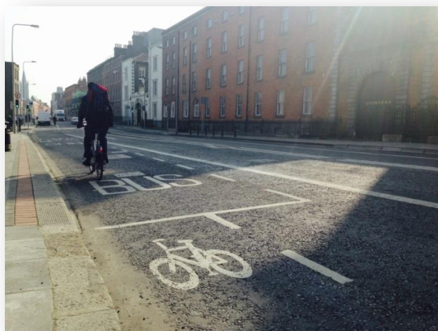
Cyclist using new facilities at James’s Street
