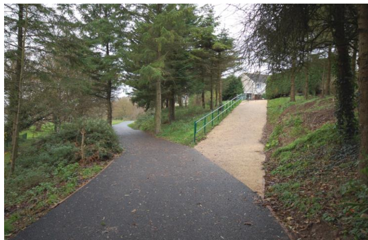
Widened and resurfaced path with cycle-friendly ramp
