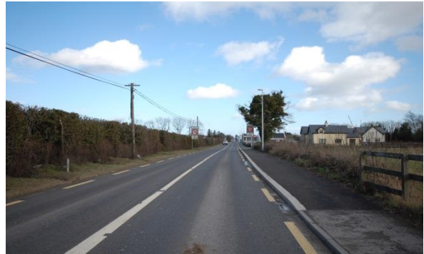
Allenwood Road (after)
