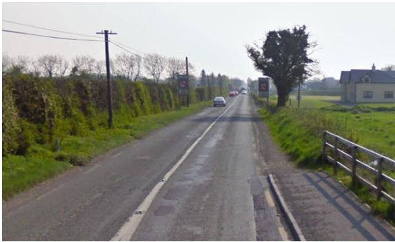
Allenwood Road (before)
