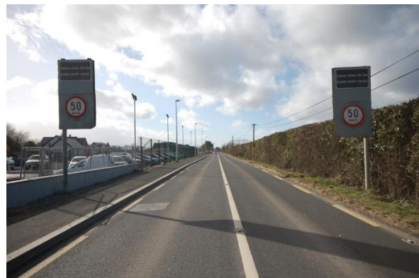
Allenwood Road (after)
