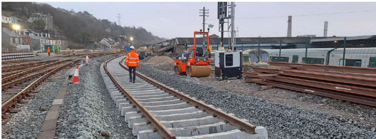
Kent station platform construction
