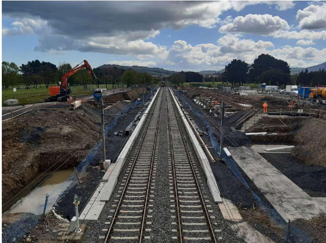
Woodbrook Station Construction Works
