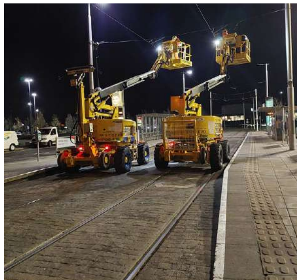
Overhead line replacement
