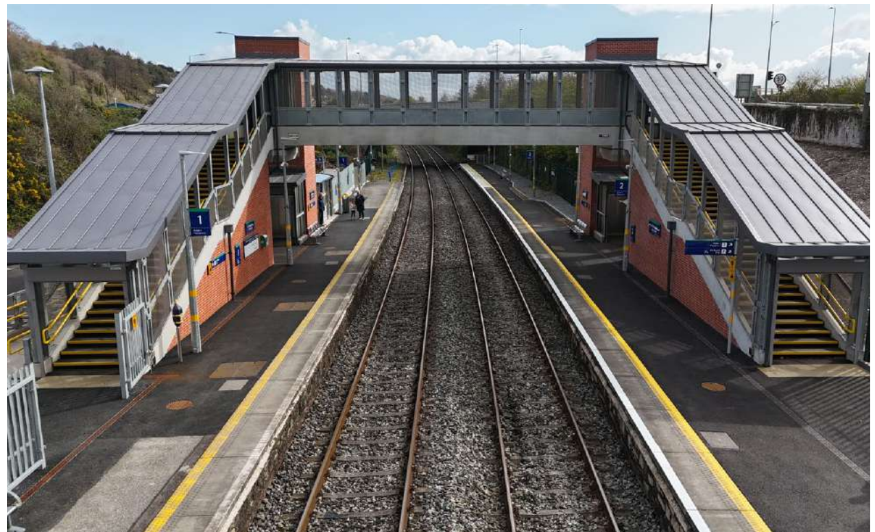
New Lifts and accessible bridge at Little Island Co. Cork
