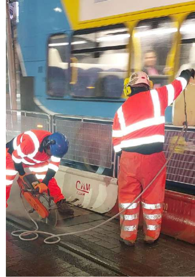
Enhancement works underway on O'Connell Street
